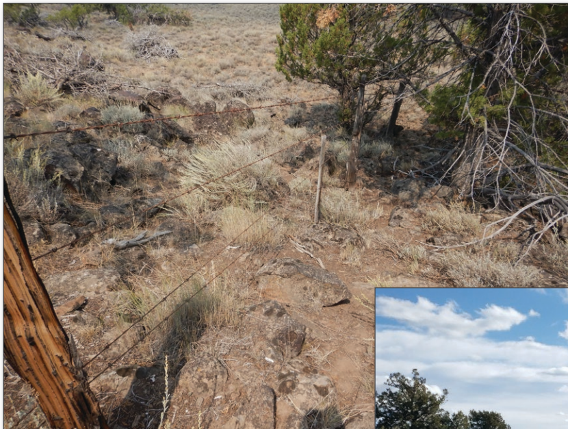
Original Fence Design (left): Barbed wire fences with a bottom wire below 16 inches can be a barrier to migrating ungulates by obstructing movements and may cause injuries to pronghorn and mule deer. This type of fence design can trap legs or snag hides, leading to stress, physical harm, and lead to mortality in some cases.
