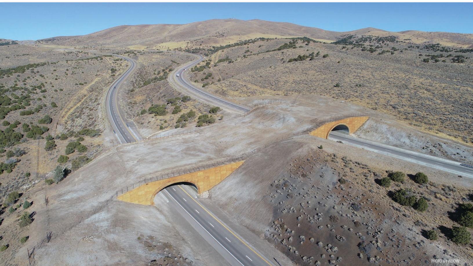
Pequop Wildlife Overpass: Beginning in 2015, planning for wildlife overpasses and modified underpasses on I-80, 18 miles east of Wells, Nevada, aimed to protect migrating mule deer and other wildlife. GPS collar and crash data identified the Pequop Summit corridor, where 60–80 deer were hit annually. The wildlife overpass and new fencing at several underpasses was completed in 2019, reducing wildlife-vehicle collisions by an estimated 90%.
